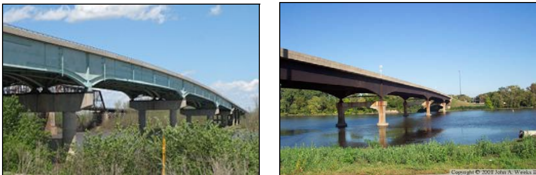
Figure 9: Lewis Bridge, 1979 (left) and Moline-Arsenal Bridge, 1982 (right)
