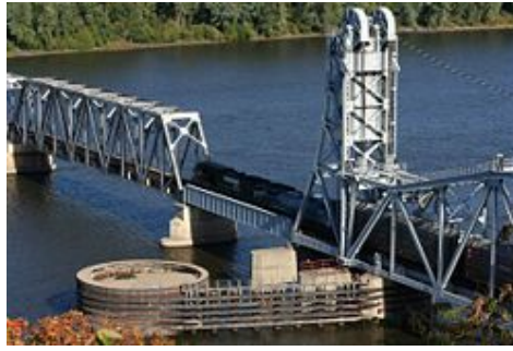
The Wabash Bridge looking southeast
